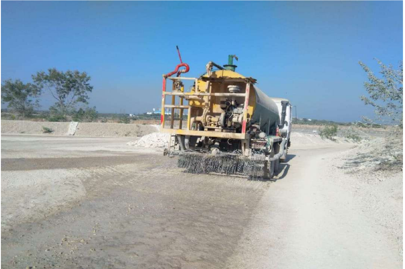
Haul Road wetting with water tanker
