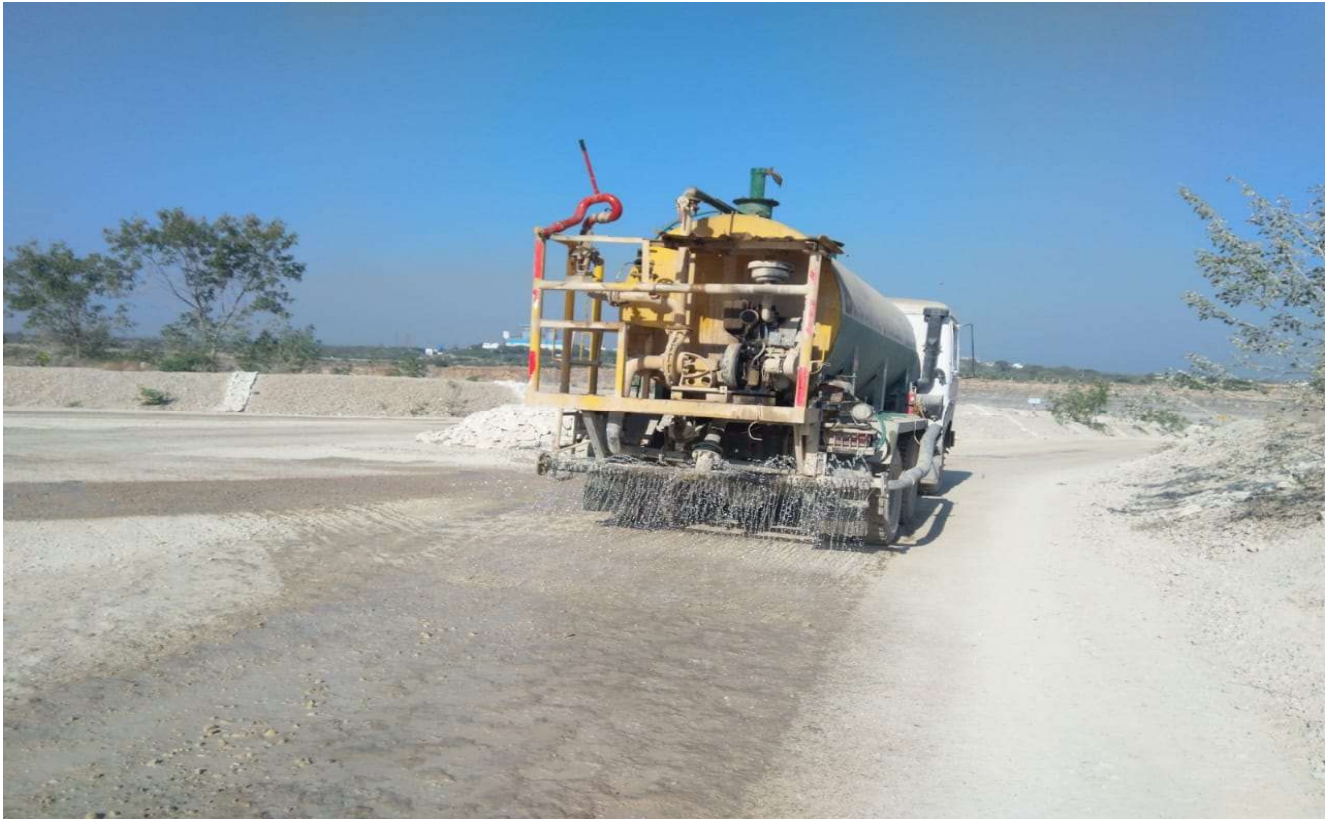
Water Sprinkling with Tanker for Dust Suppression.
