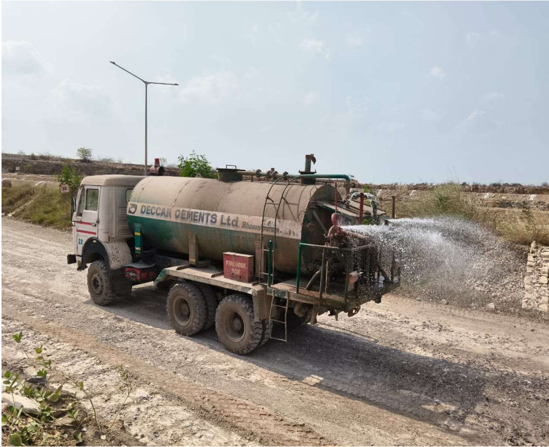
Haul Road wetting with water tanker
