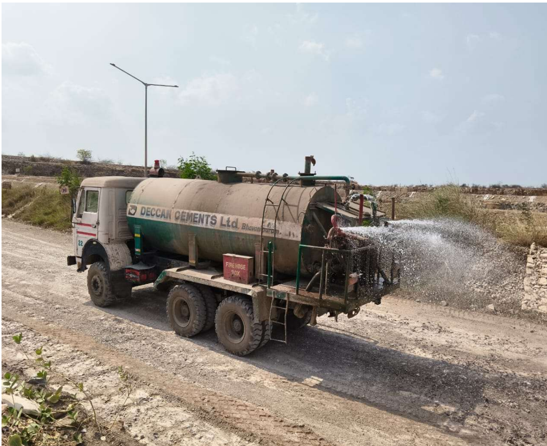
Water Sprinkling with Tanker for Dust Suppression.
