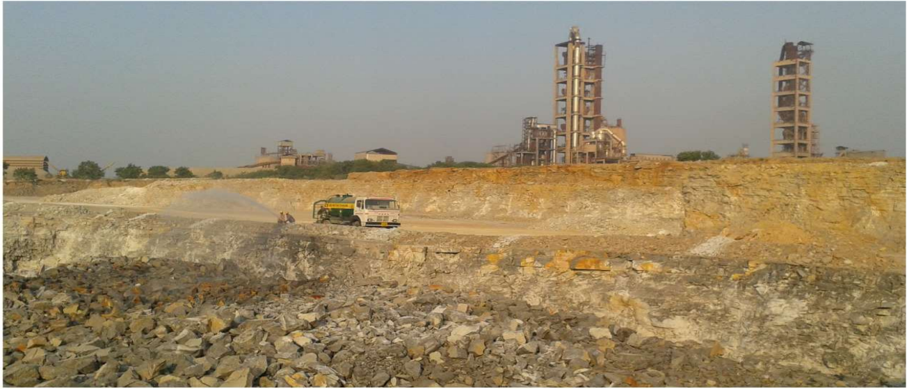
Wetting of Blasted muck pile before loading to reduce dust generation
