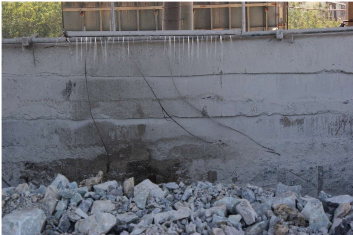
Water Spray at Crusher Hopper
