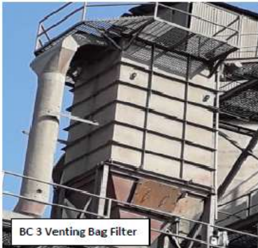
Cement Mill-1&2 Mill venting Bag House
