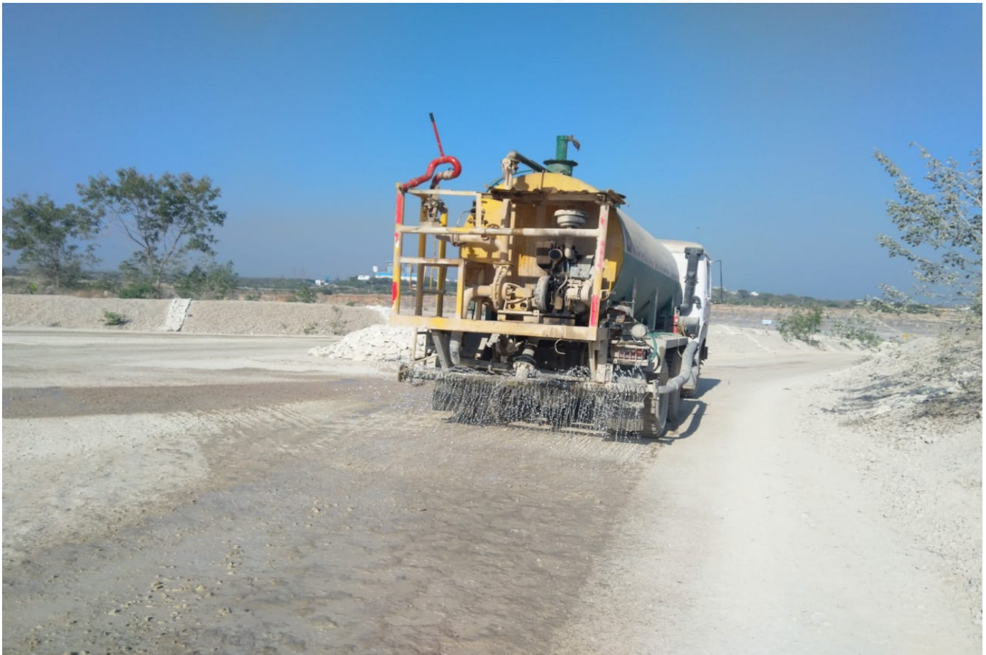
Haul Road wetting with water tanker
