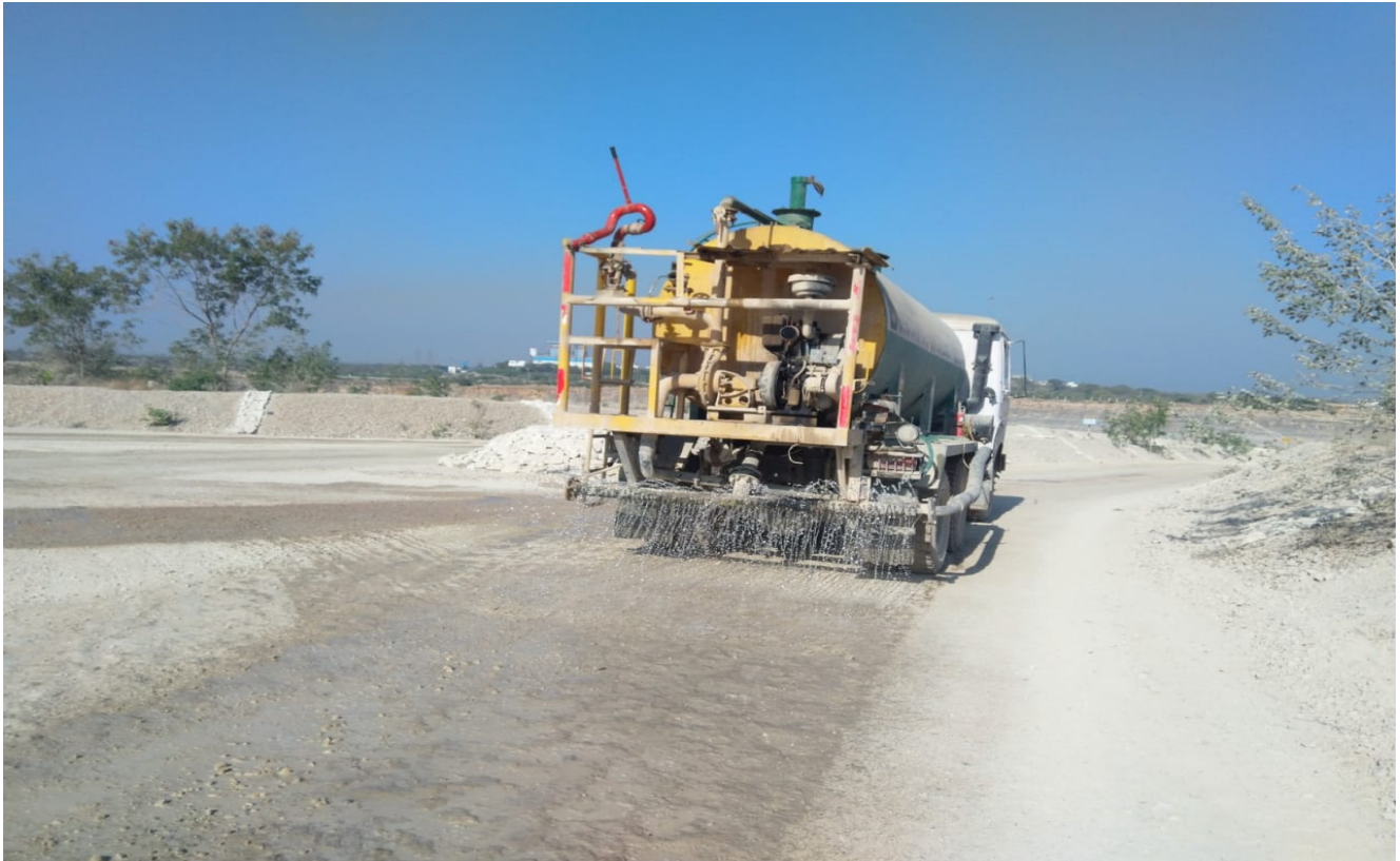
Water Sprinkling with Tanker for Dust Suppression.
